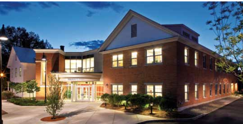
The new Keene State College Alumni Center, dedicated on Reunion Weekend in June, provides space for alumni meetings and social gatherings, career mentoring, intergenerational programs, and community-building activities. It houses the Advancement division offices, including Alumni and Parent Relations, Development, Marketing & Communications, and Advancement Services.
